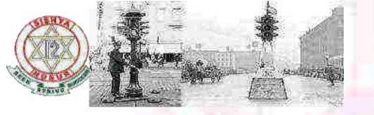
On August 5, 1914, the world's first electric traffic signal was installed to the corner of Euclid Avenue and East 105th Street in Cleveland, Ohio. It was designed by James Hoge and patented in 1918. The first traffic signal comprised of four pairs of red and green lights that served as stop-go indicators, each mounted on a corner post.
